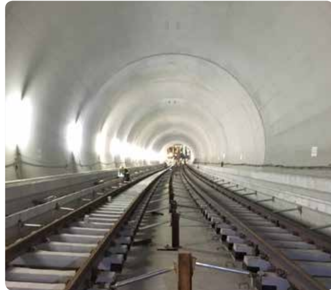
Nishiya Tunnel on the Through Line between Sotetsu and JR
