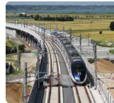
Narita Rapid Rail Access Line (Narita Sky Access Line) ● Awards: Japan Society of Civil Engineers Outstanding Civil Engineering Achievement Award (2010), others
