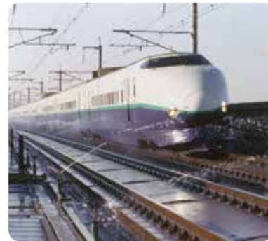
Joetsu Shinkansen ● Awards: Japan Society of Civil Engineers Outstanding Civil Engineering Achievement Award (1980), others
