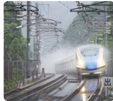
Hokuriku Shinkansen ● Awards: Japan Society of Civil Engineers Outstanding Civil Engineering Achievement Award (2015), others
