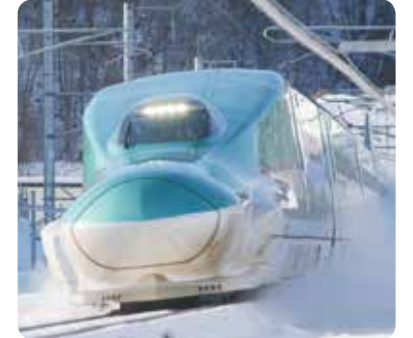
Hokkaido Shinkansen ● Awards: Japan Society of Civil Engineers Outstanding Civil Engineering Achievement Award (2012), others
