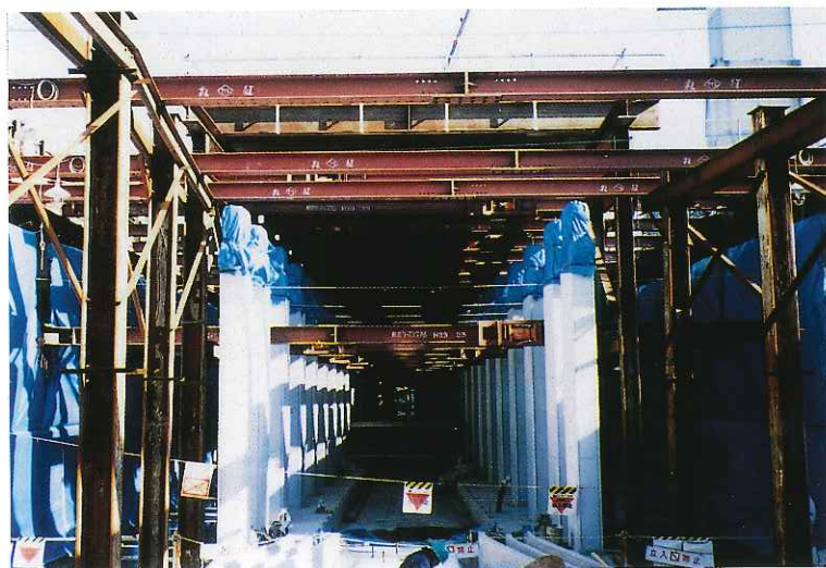
T2工区く体構築
