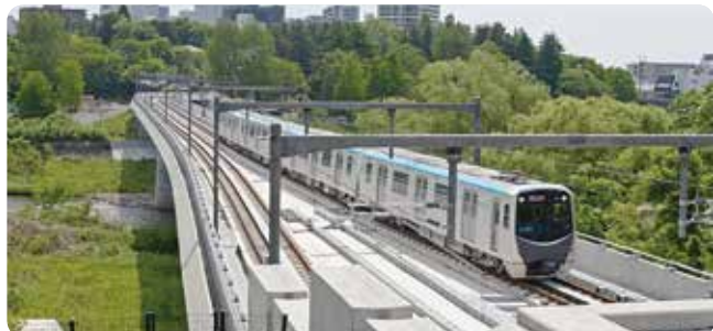
Subway construction (Sendai Subway Tozai Line) Photo provided by the Sendai City Transportation Bureau
