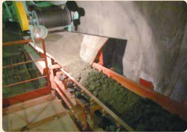
Earth and sand removal by belt conveyor inside a shaft
