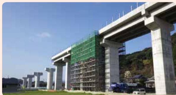
Hakamano Bridge in Saga Prefecture
