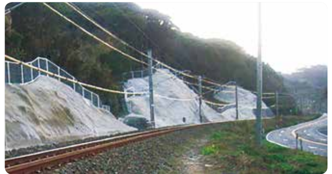
Railway disaster prevention work: Rockfall prevention measures (Kyushu Railway Company)
