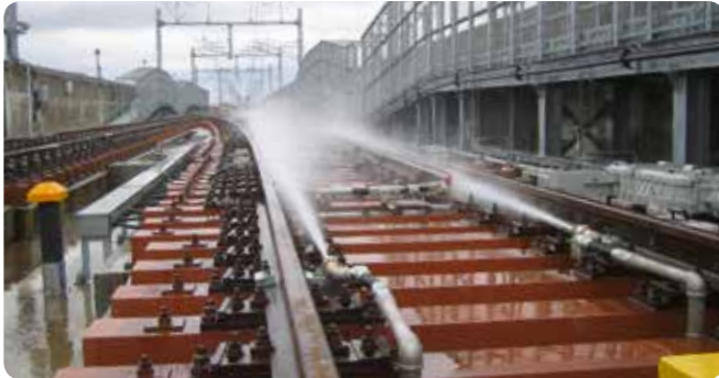
Air-type rapid snow removal equipment Equipment that rapidly removes snow that falls from rolling stock onto point frogs (Hokkaido Shinkansen)
