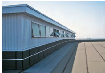
Natural ventilation systems, green roofs at Hakusan General Rolling Stock Depot, Hokuriku Shinkansen
