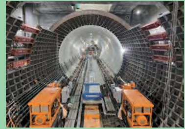
10 Sasson Tunnel (launching shaft)
