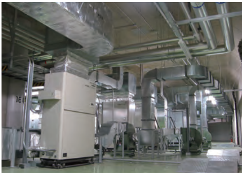
Air conditioner in underground station
