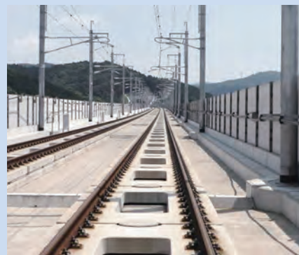
Frame type slab (Kyushu Shinkansen)
