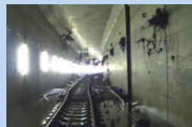
Inside the airport tunnel
