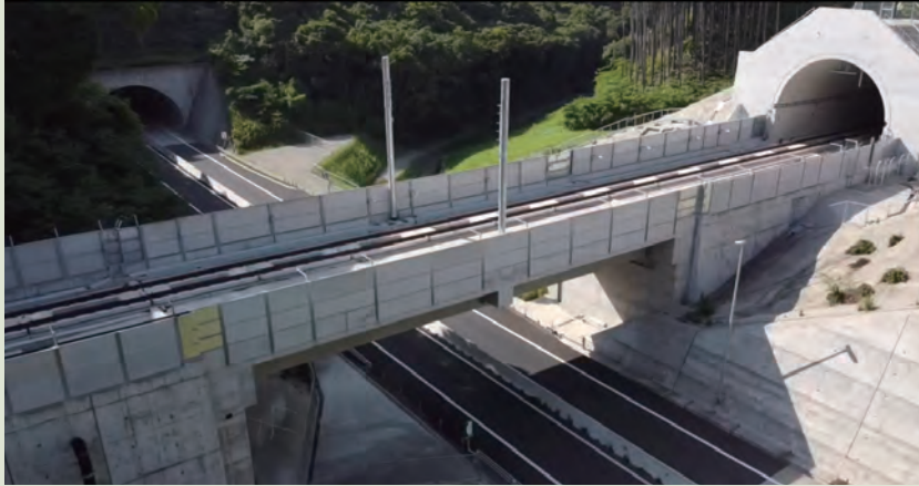
Genshu Bridge (GRS-integrated bridge with PC girder) Kyushu Shinkansen
