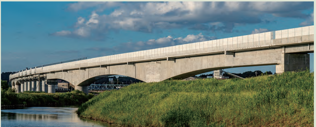
No.2 Takeda River Bridge Hokuriku Shinkansen
