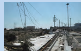
Entrance to the airport tunnel
