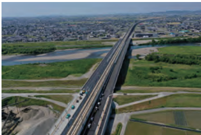
9 Kuzuryu River Bridge
