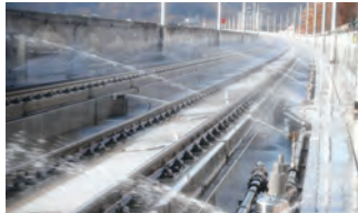
Snow removal sprinklers
