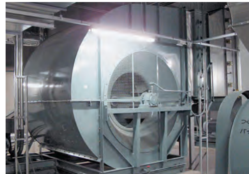
Ventilator for tunnel
