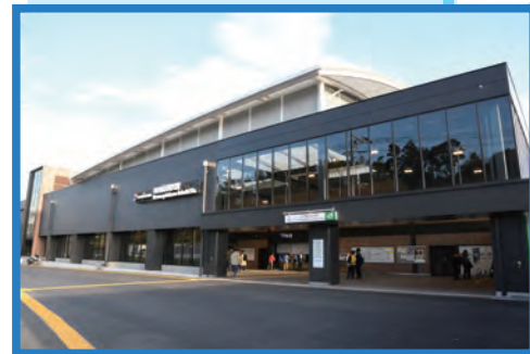
3 Hazawa yokohama-kokudai Station
