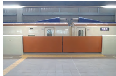
Screen door on the platform
