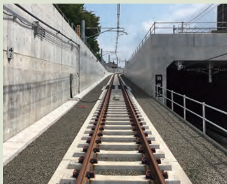
Ballastless track with solid bed track with resilient sleepers (Sotetsu-JR Link Line)
