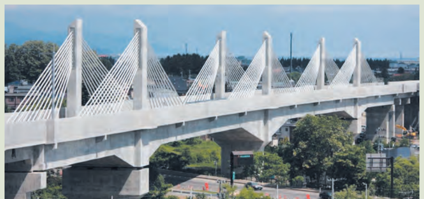
Sannai-Maruyama Bridge, Tohoku Shinkansen
