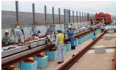
Construction of rail track
