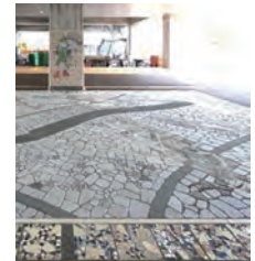
Use of recycled tiles at Narita Yukawa Station, Narita Sky Access Line
