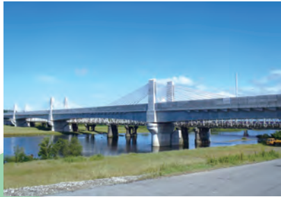
4 Jinzu River Bridge
