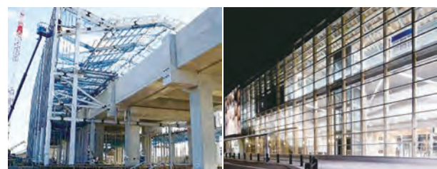
Shin-Tamana Station, Kyushu Shinkansen The architectural exterior completely covers its civil engineering structure.
