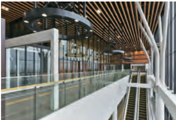
Louver ceiling made of locally sourced wood at Shin-Hakodate Hokuto Station, Hokkaido Shinkansen
