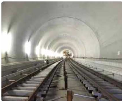
Nishiya Tunnel on the Through Line between Sotetsu and JR
