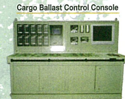
Cargo Ballast Control Console
