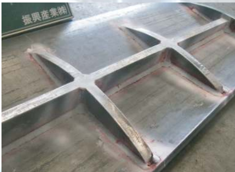
③ 溶接及び浸透探傷検査 Welding and PI
