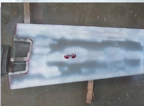
⑤ 溶接及び浸透探傷検査 Welding and PI
